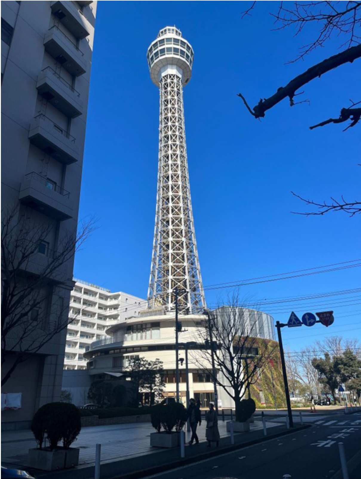
Figure 1 - Photo of the Yokohama Marine Tower Source: Taken by the author in January 2023.
